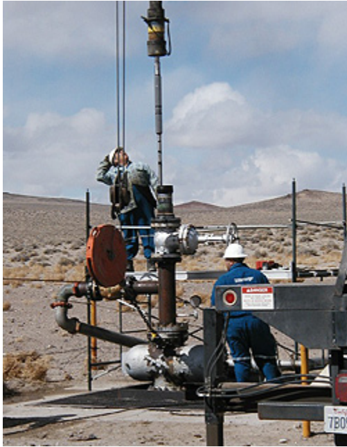
Drilling of a geothermal exploration well at the Desert Peak site in Nevada. National Renewable Energy Laboratory
